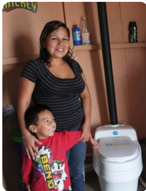
Customer Gloria Canchaya has just had her new toilet installed by Sanima. She is one of 3.000 customers who have been provided by Sanima.
